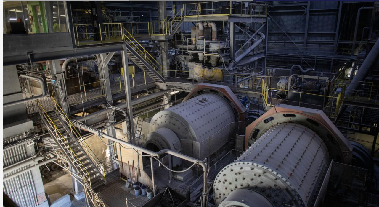
Empire State Mine Processing Facility
