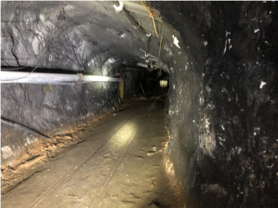
Figure 5 – 1,500-Foot Tramway in Good Shape on 2500 Level at #2 Mine; Connects #2D Zone to an Existing Ore Pass to the Underground Crusher at the Bottom of #4 Shaft
